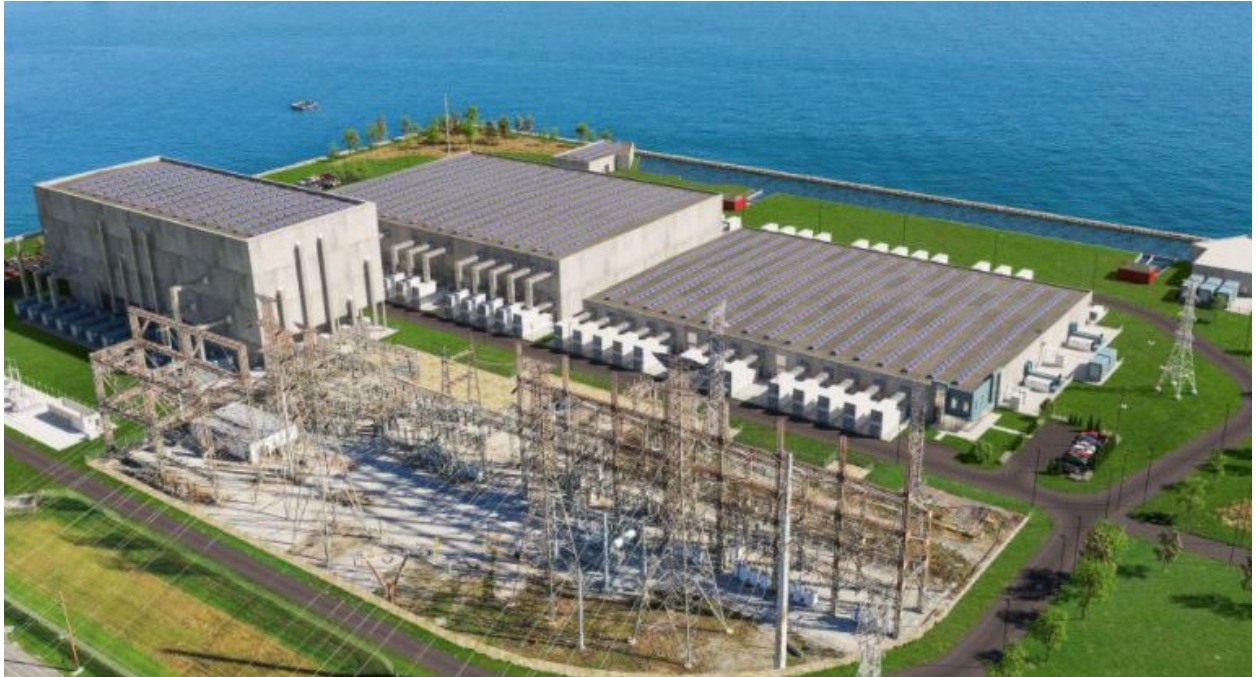
Digital Crossroads Data Center in Hammond, Indiana.
